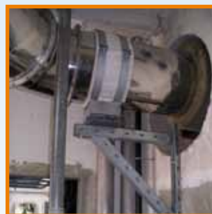
Support with MPT channel supports and MPT consoles
