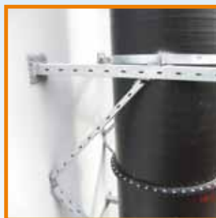
Pipe support with additional fixation
