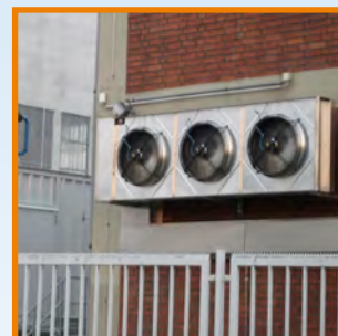
External mount of air conditione
